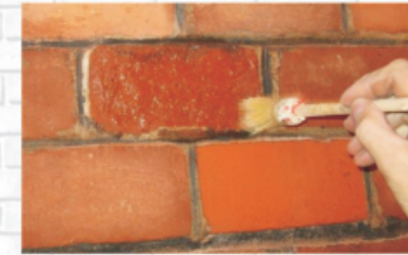
The sandstone hardener is applied with a brush
