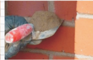
The rehabilitation pointing mortar is applied with a trowel
